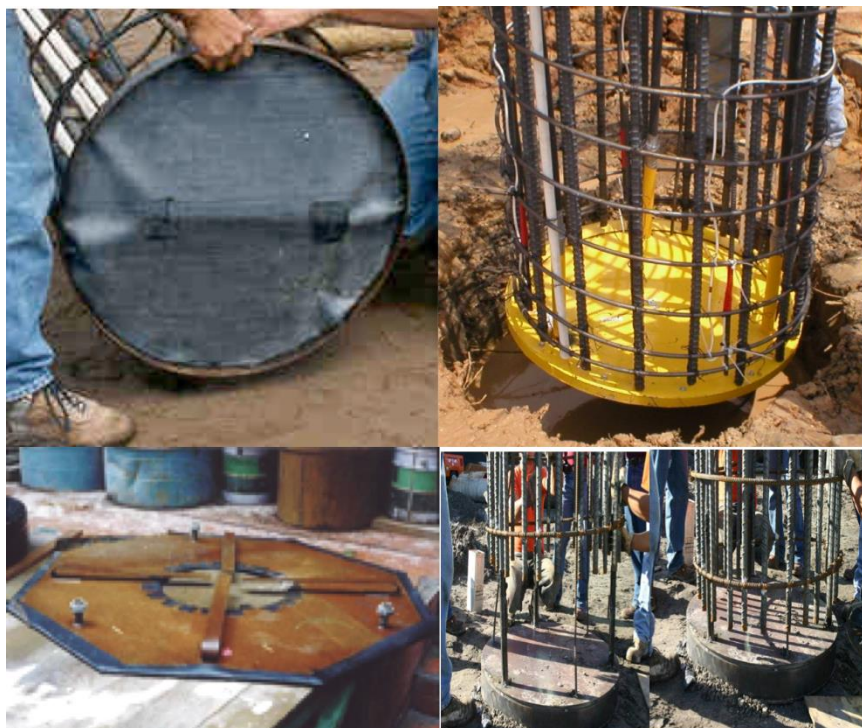
Figure 2.1 Flat jacks used in West Palm, FL (top left), Houston, TX (top right), Taipei, Taiwan (bot left), and Tampa, FL (bot right).
